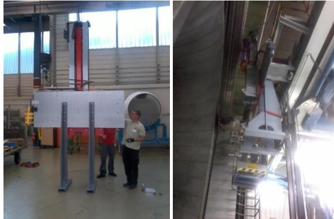
**Figure 6.3. Installation of the y-z traversable probe; (left) attachment of probe to the jigs for the installation with the forklift; (right) installation of the probe in the test cell.**
