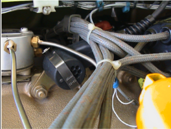
C) Installation of RPM sensor, independent from A/C electrical system, at main hook of engine, behind fuel divider (experience from HBKEZ)
