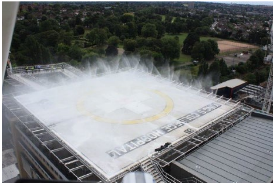
Figure II-6-5. A foam DIFFS on a solid plate surface at an elevated heliport
