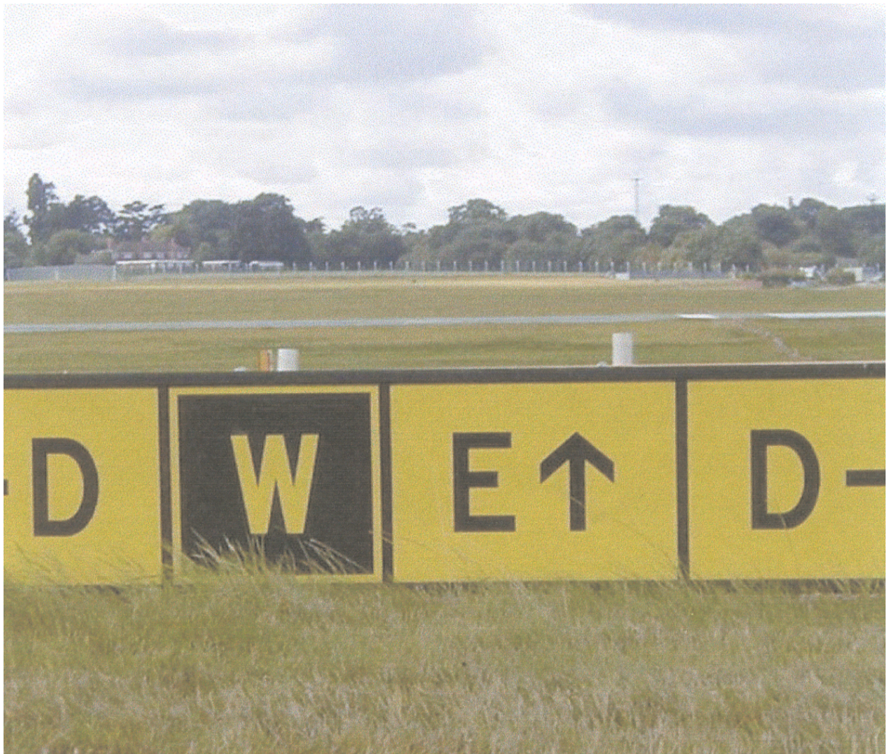
Figure 12-1. Example of a complex sign layout
